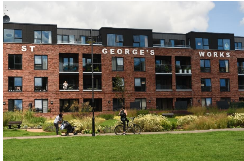
St George's Works development, Trowbridge
