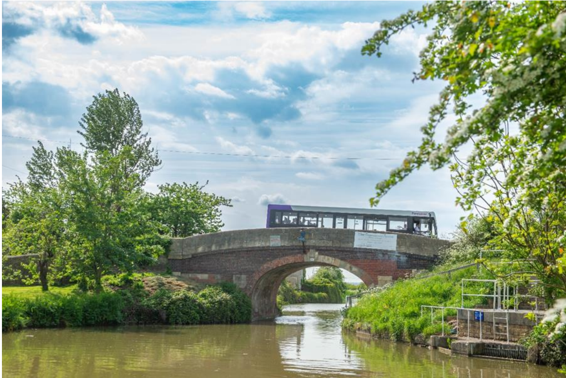
Semington Road Bridge, over the Kennet and Avon Canal
